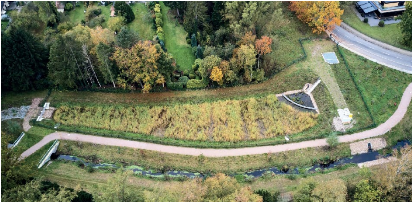
Figure 4: Constructed wetland for the treatment of a stormwater catchment in Hamburg. Source: HAMBURG WASSER.
