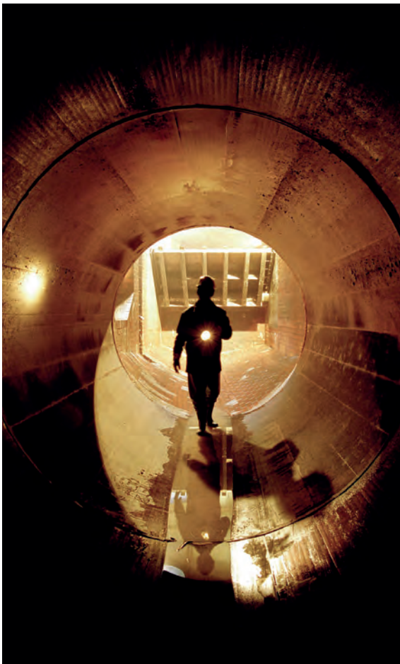
Picture: A view through a storm relief sewer with the weir of the sewage flow diverter in the background
